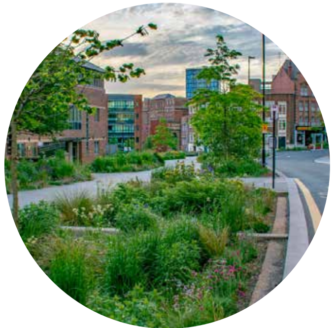
18. Example of Sustainable Drainage System in Sheffield
